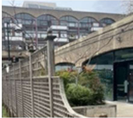
Remove wooden fencing from tennis courts, create a green wall and replace the alleyway.
