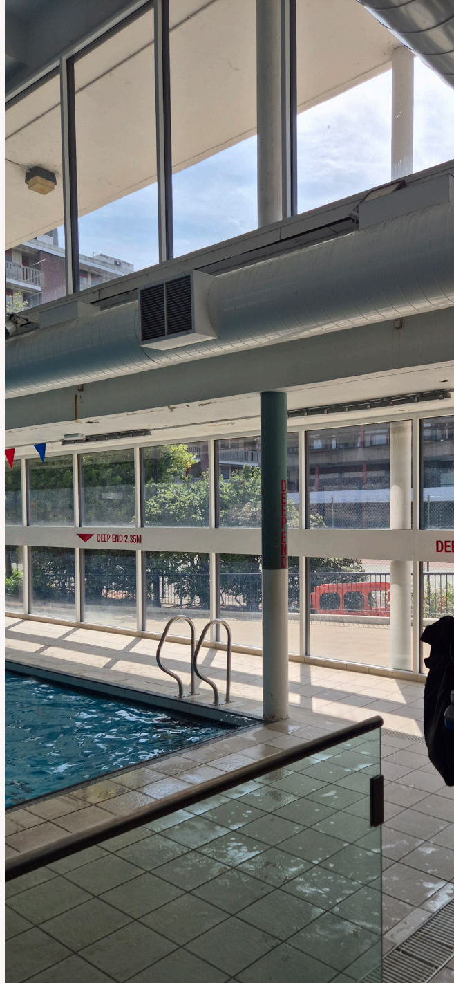
Existing Building - Internal
