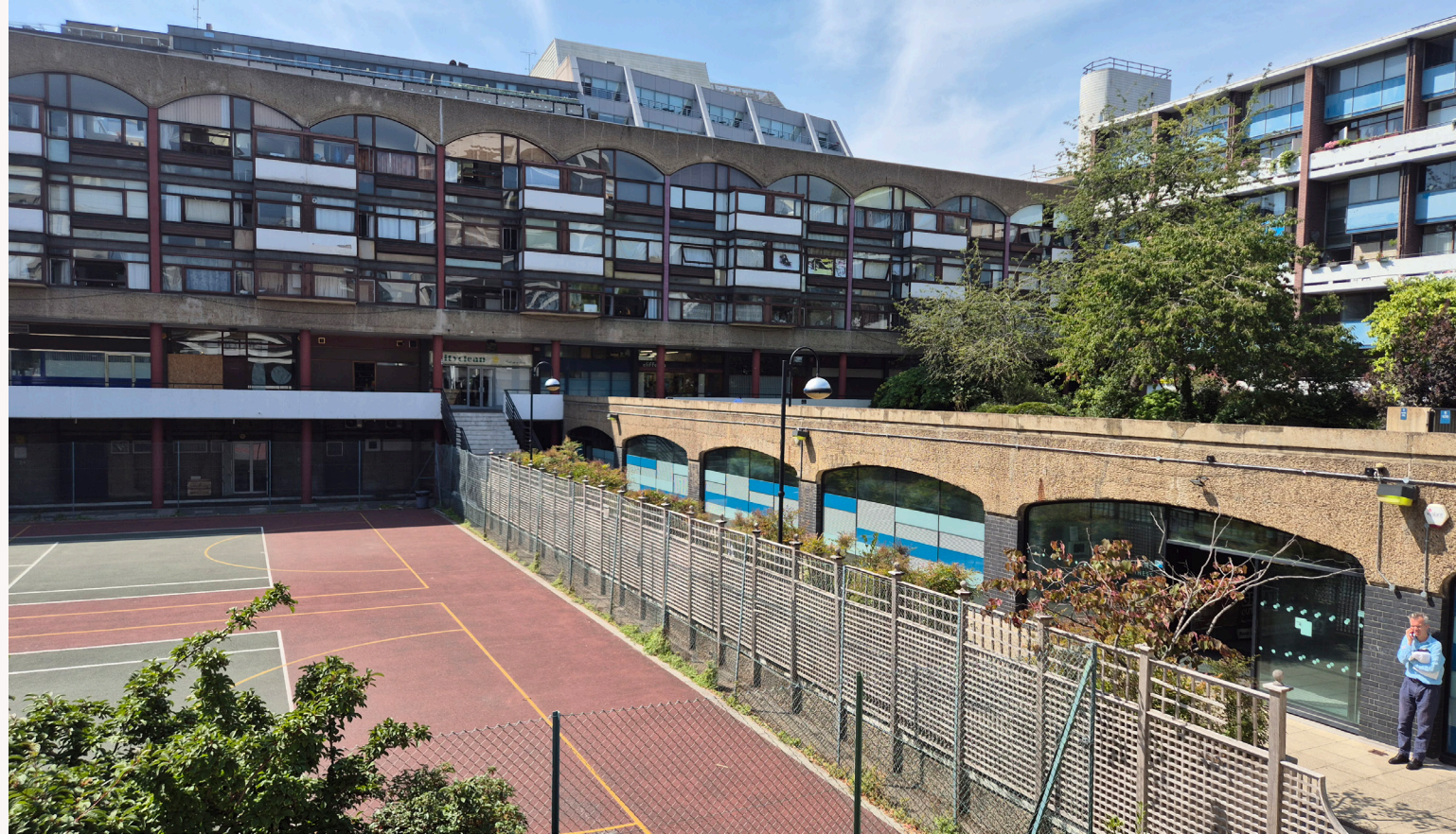
Existing Building - External
