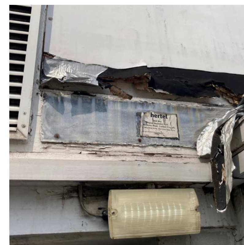
Tank room enclosures
