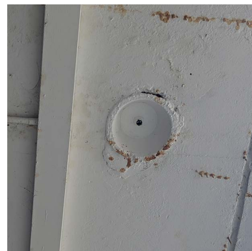
Redundant recess for original lighting at Crescent House
