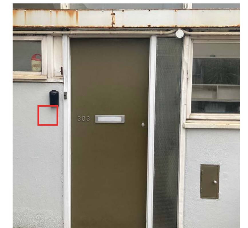
An example of where soffit mounted lighting to a front entrance door is not possible.
