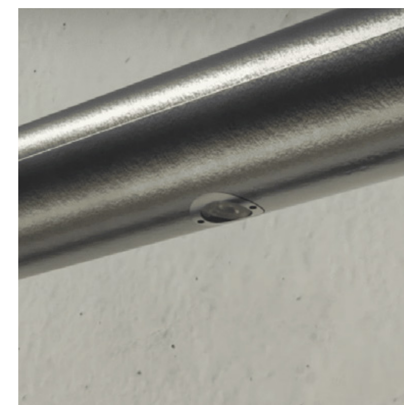
Lighting recessed into handrails
