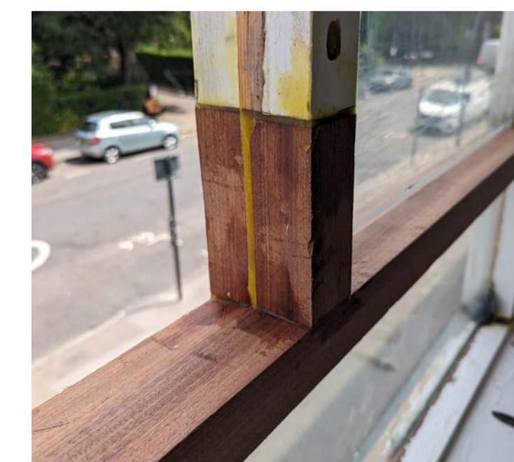
Example of replacement (and splice) repair carried out in Stanley Cohen
