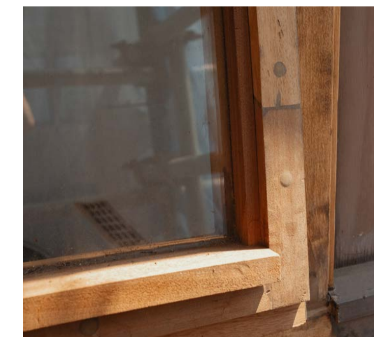
Example of splice repair carried out in Crescent House
