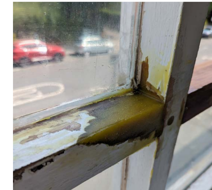
Example of resin repair carried out in Stanley Cohen
