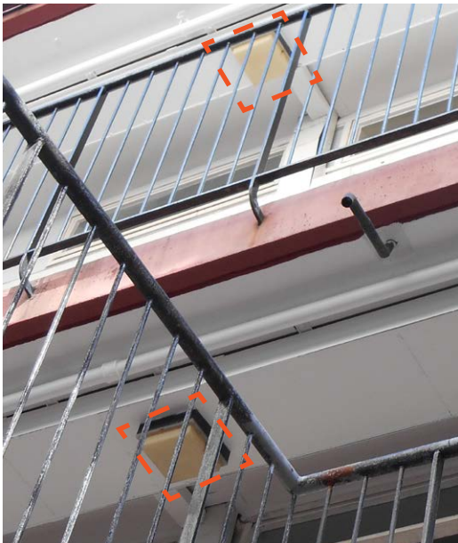
View looking into upper floors of Crescent House (courtyard). Fittings cat. 2.
