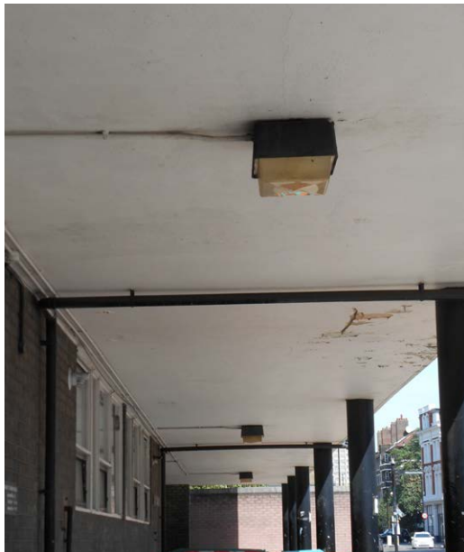
16 Stanley Cohen House (Golden Lane) - View looking north. Fitting cat. 2.
