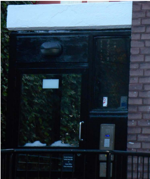
Lights in front of Hatfield House. Fittings cat. 10.
