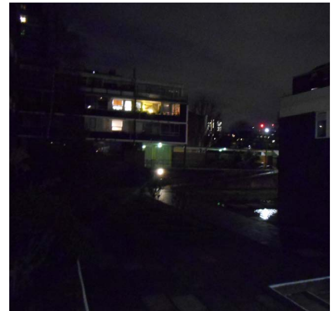
⑥ View looking into Pond Area.
