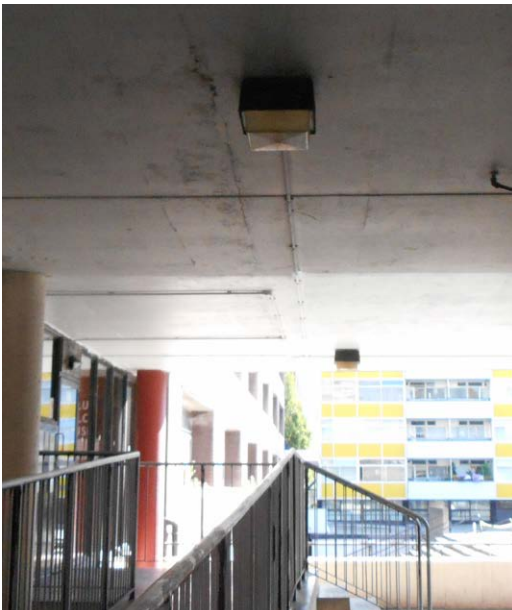
View looking in to plaza from Goswell Road. Fitting cat. 2.
