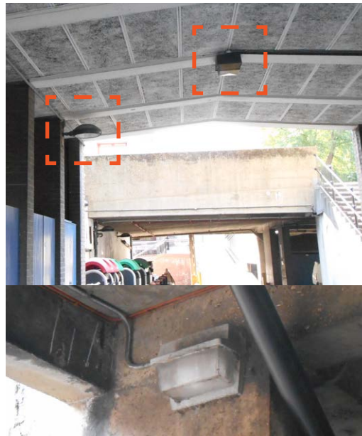
View looking south into refuse area. Fittings cat. 2 and cat 22.
