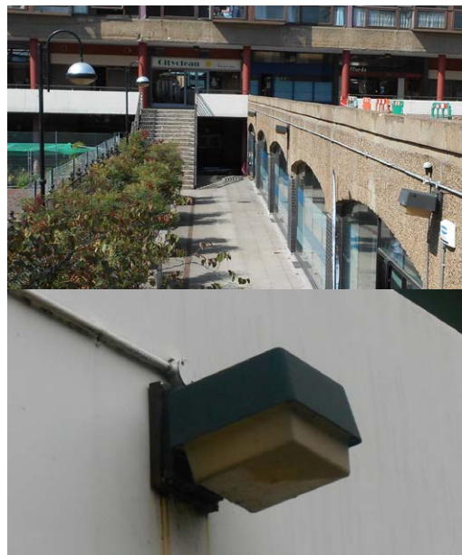
View looking into Golden Lane Day Nursery, City Walkway lights. Fittings cat. 3 and cat. 14.
