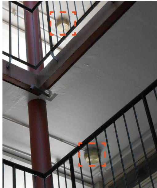
View looking into upper floors of Crescent House (courtyard). Fittings cat. 1.
