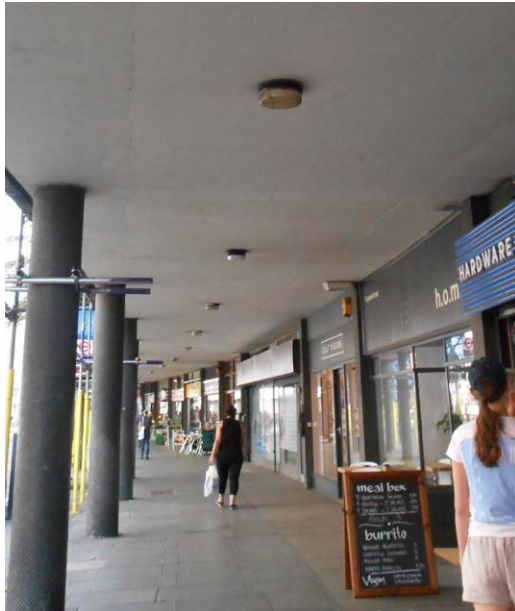
View looking north of Crescent House. Fitting cat.1.
