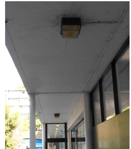
View looking north into swimming pool. Fittings cat 2.
