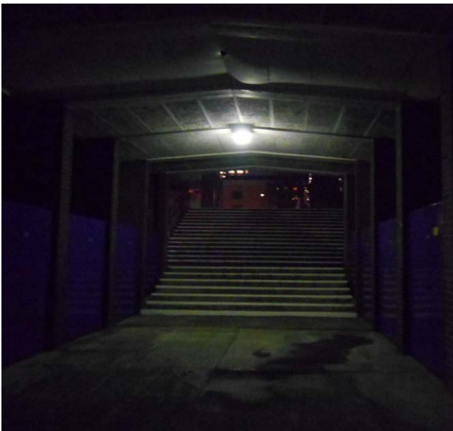
④ Storage area under Collum Welch House looking into stairs leading to plaza.
