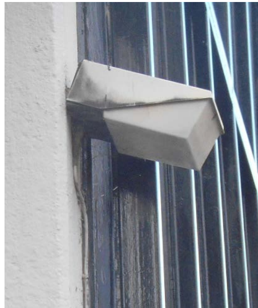
External fittings on Cuthbert Harrowing House. Cat. 16.
