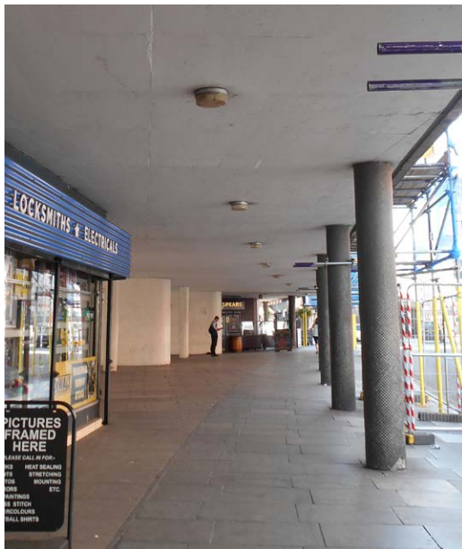
View looking south of Crescent House. Fitting cat.1.
