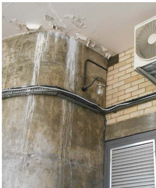
Garage lighting. Fittings cat. 6. (Assumed as original fitting.)
